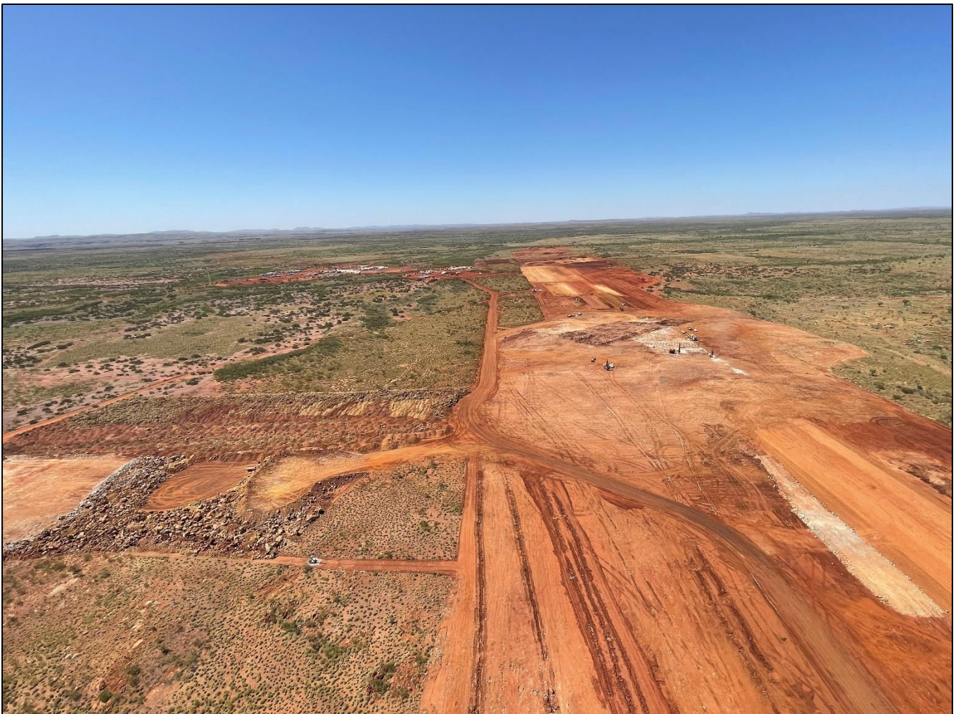
Figure 2 – Construction of the RHIOJV Airstrip and Camp.
